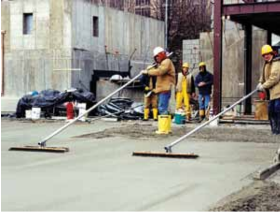
Fig. 3: Workers broom a slab-on-ground. Vulnerability to rain damage depends on when the rain event occurs relative to the setting time as well as the intensity of the downpour. Workers should avoid finishing additional water into the slab
