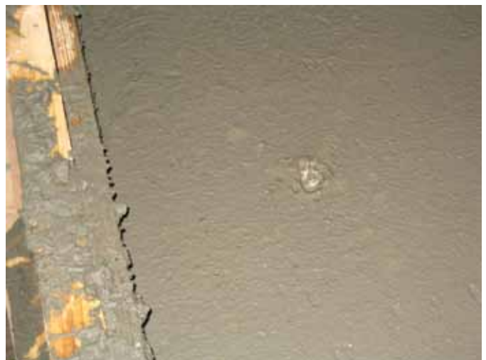
Fig. 1: View of the effect of drops of rainwater on fresh concrete
