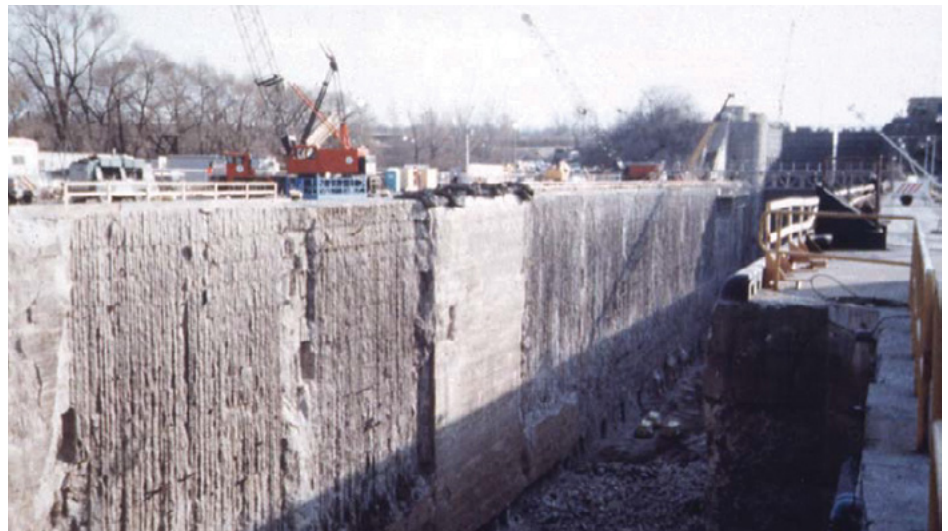
Fig. 1 Close-line drilling along with explosive charges in alternating drill holes was used to remove deteriorated lock walls during rehabilitation.
