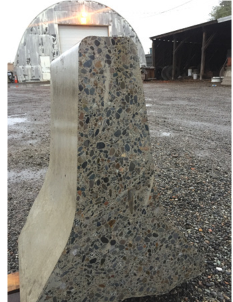
Fig.3a Traffic barrier saw cut to provide visual examination of its cross-section.
