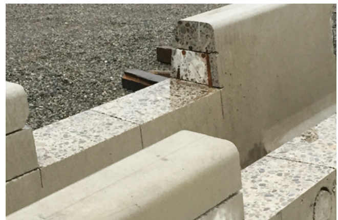
Fig. 3b Slices through traffic barrier exhibit uniform aggregate distribution and good consolidation around reinforcing steel maintaining proper concrete cover.
