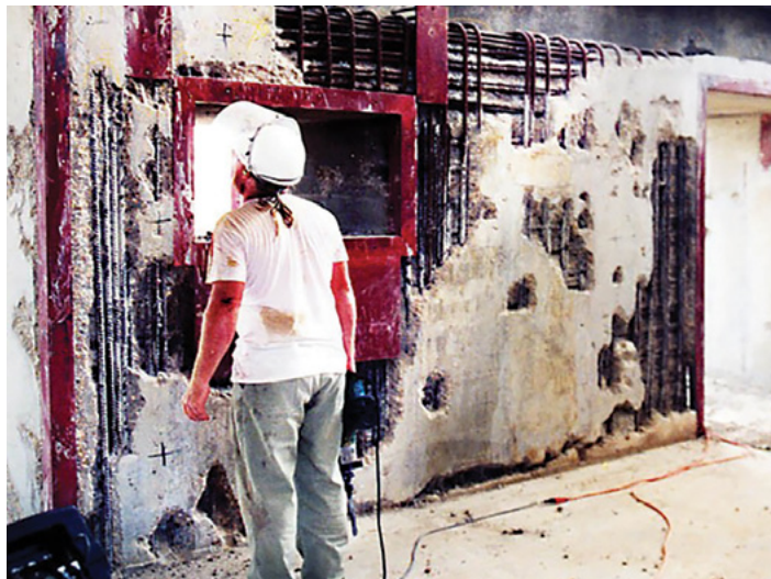
Fig. 4 Difficult conditions for concrete placement within forms and deficient consolidation in highly congested foundation.
