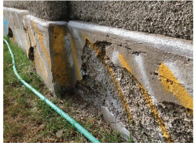
Fig. 1—(left) Cemetery maintenance of walls consisted of mortar application over cracks or spalls, photo taken in September 2013; and (right) photo of pervious wall at nearby St. Boniface Cemetery in good condition.
