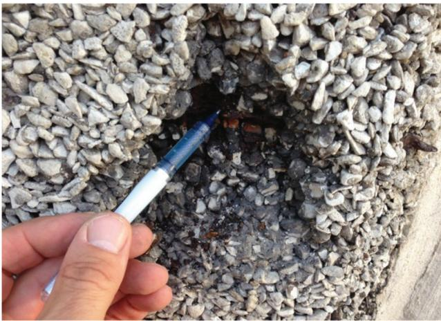
Fig. 2—Recent spall revealing corrosion products deposited in voids adjacent to steel.
